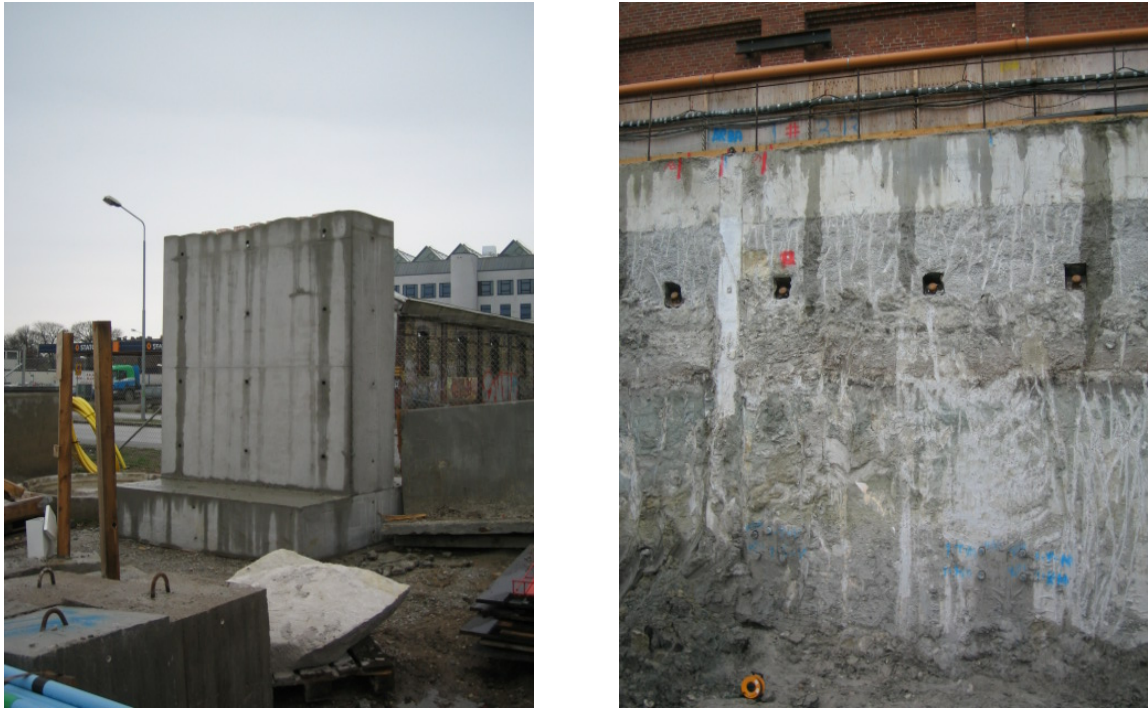
Figure 3.1: Reference panel (left) and diaphragm wall panels (right)
