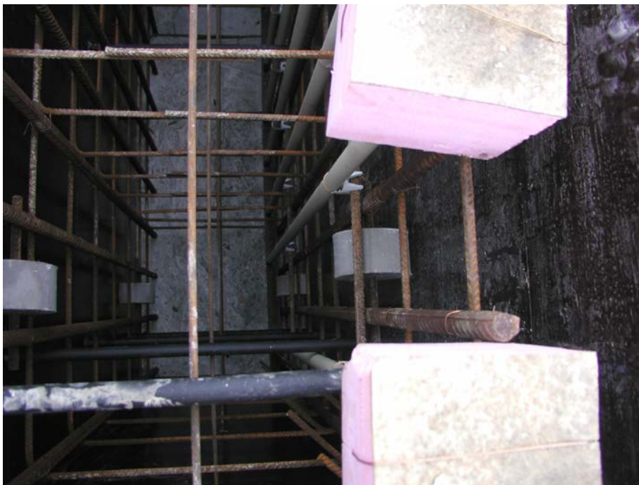
Figure A.4: Reinforcement cages and bars for pull-out tests covered with polystyrene caps in diaphragm wall panels
